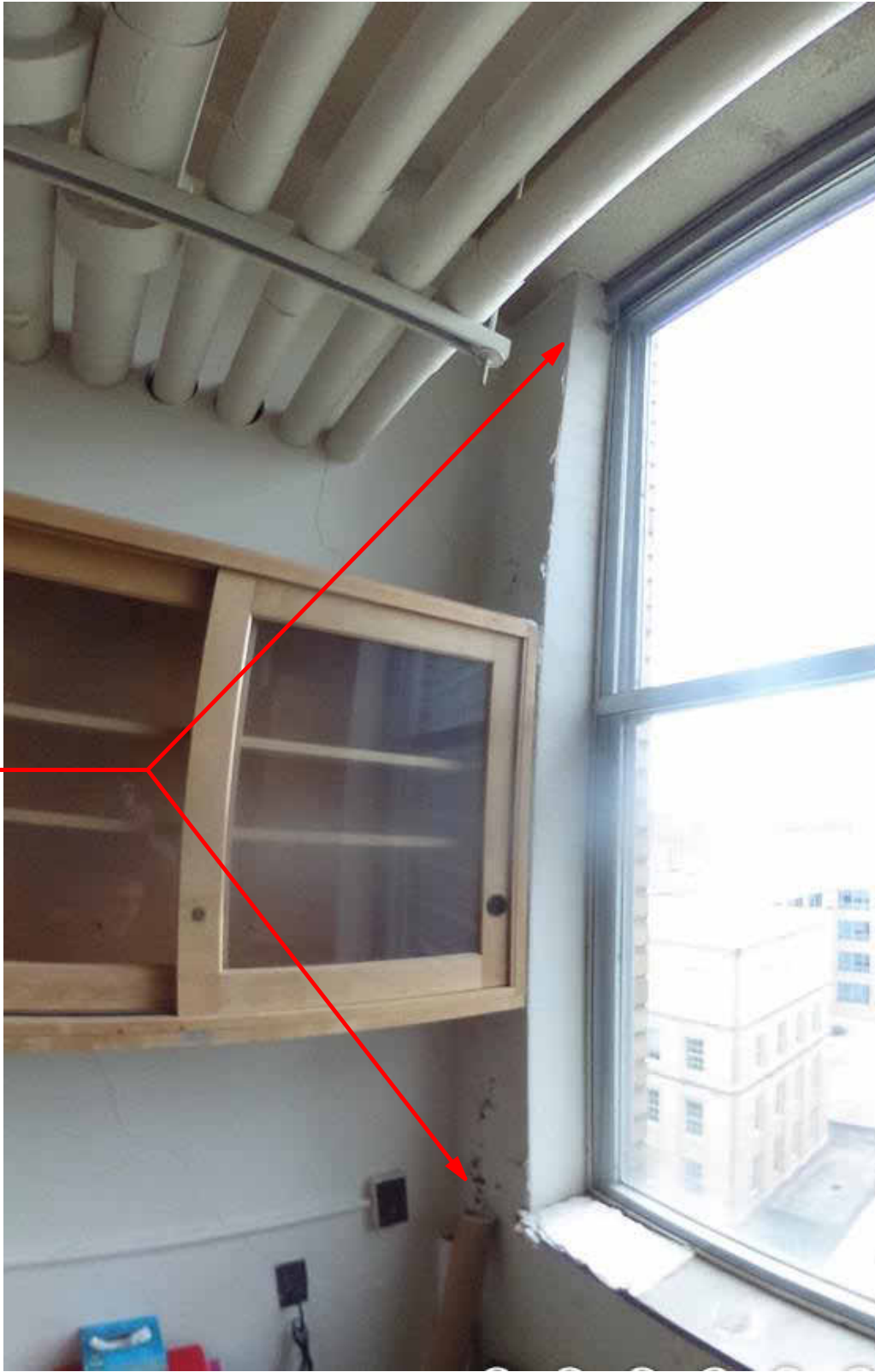
PHOTO 2: WINDOW AT SOUTH OF RESEARCH LAB 406A
