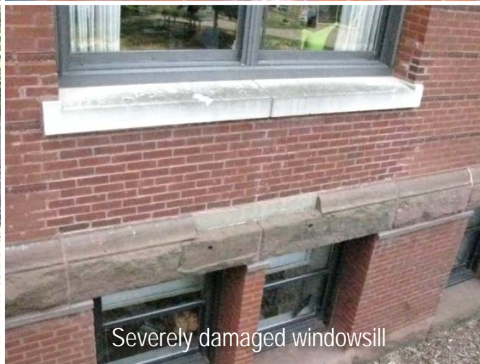
Deteriorated joints between stones
