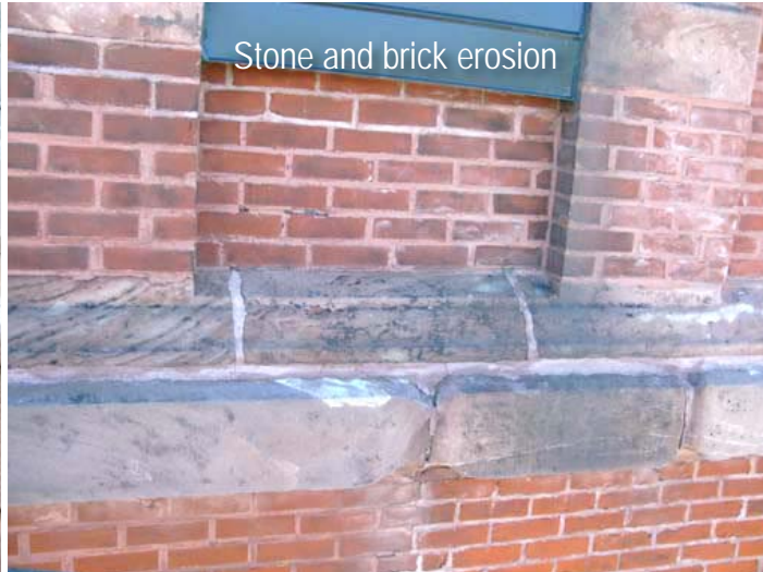
Water enters wall at sandstone band.
