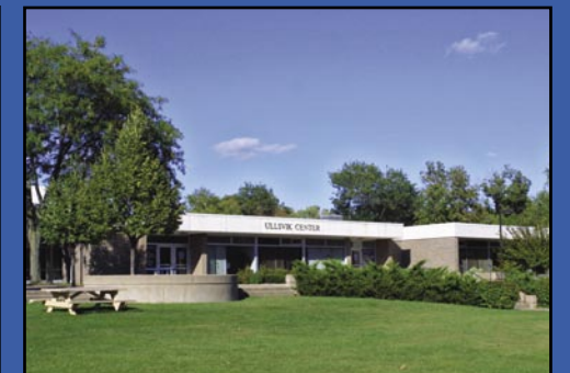
Ullsvik Center Remodeling and Addition (2005-07) GPR/PR
